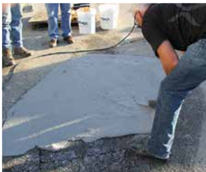
Place Elephant Armor™, folding product into precut groove
