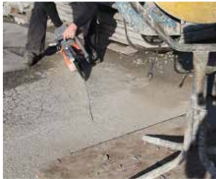
Saw cut a groove around repair to create a hard edge
