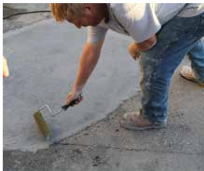
Roll surface with a texture roller to mimic asphalt appearance
