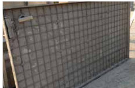
Old material is removed from panels
